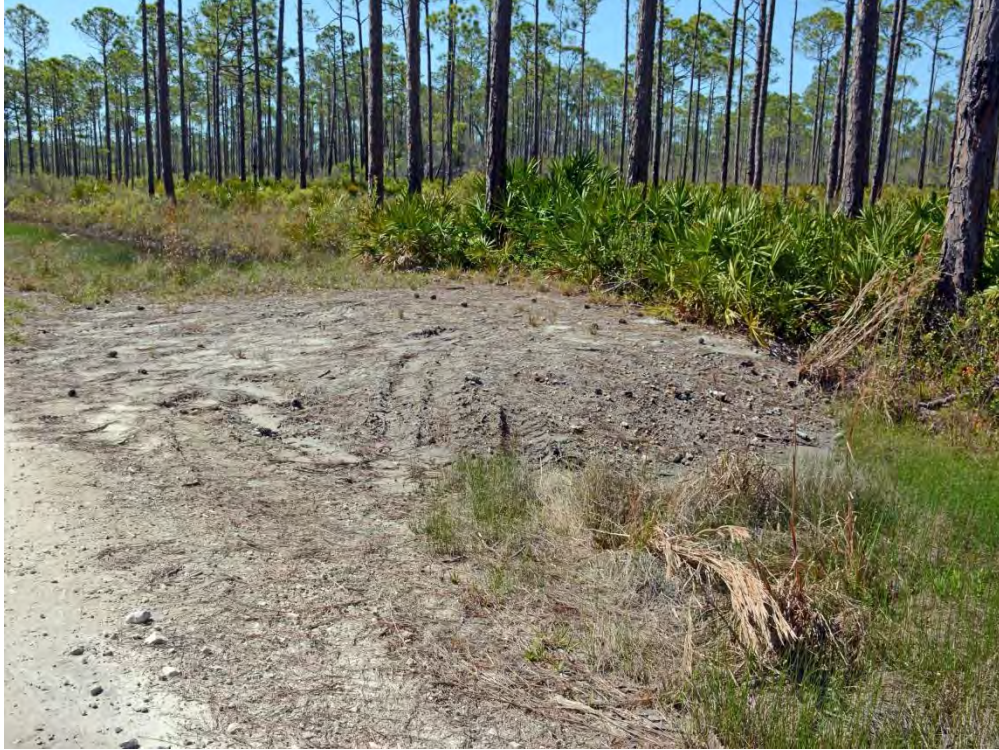
Typical Ditch Plug with Adjacent Hydric Pine Flatwoods in Background (4/19/2016)
