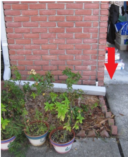
Figure 3a. Roof gutter down spout draining onto a concrete driveway
