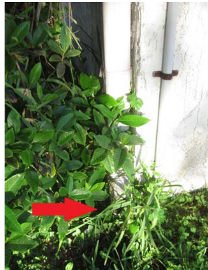
Figure 3b. Roof gutter down spout draining onto grass
