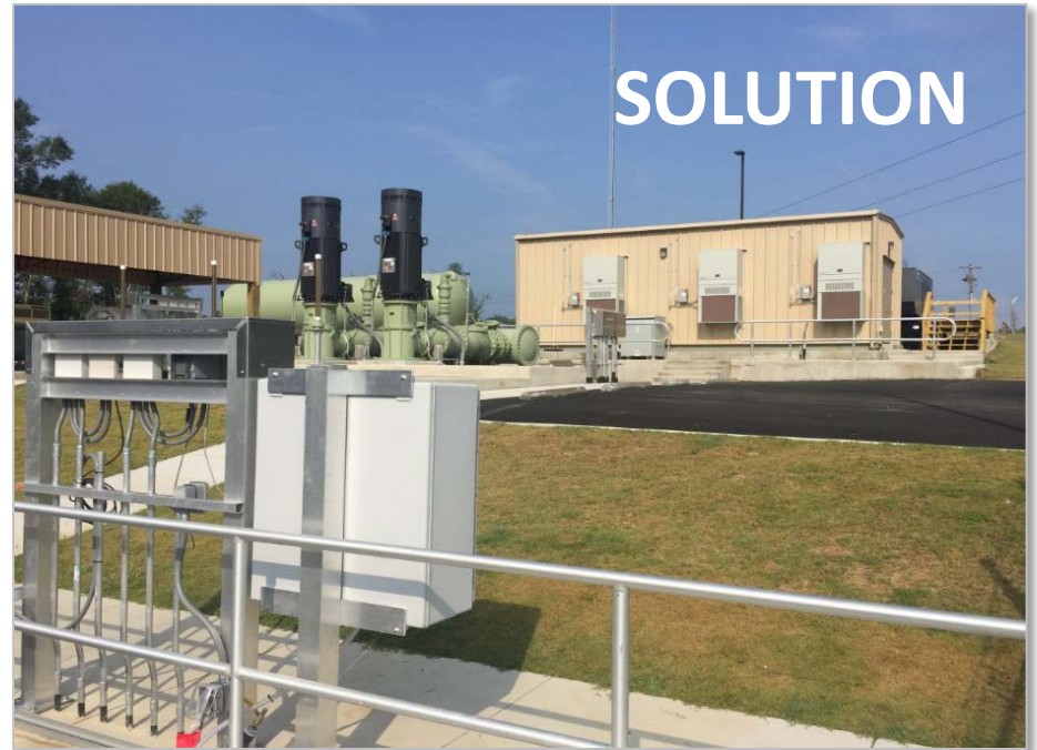
Alternative Pump Station, Econfina Creek
