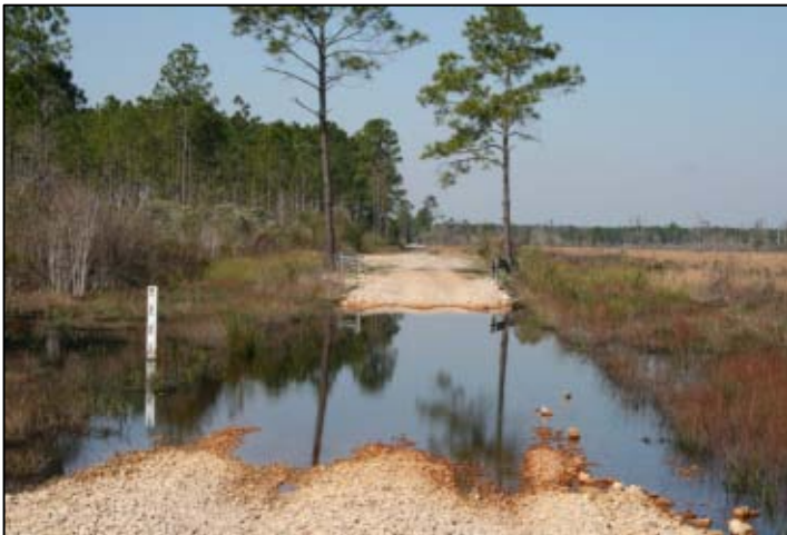
Figure 2. Low water crossing
