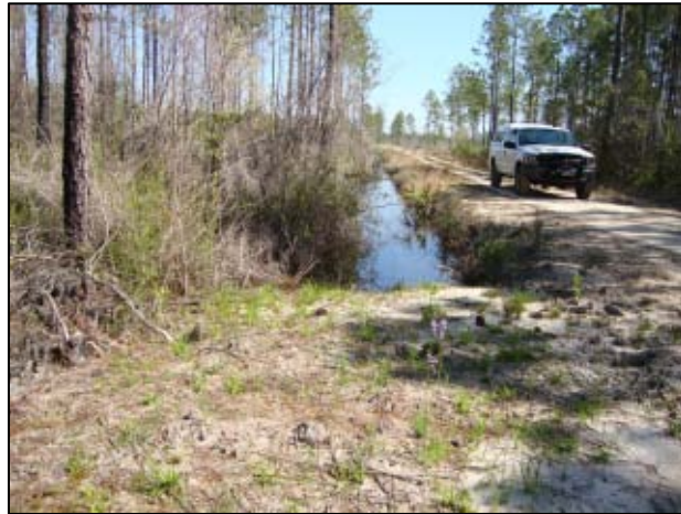
Figure 3. Earthen ditch block
