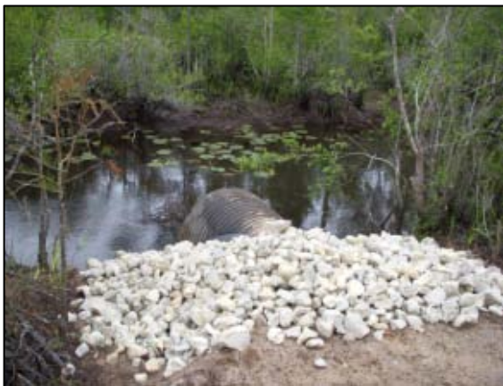
Figure 4. Recently installed culvert
