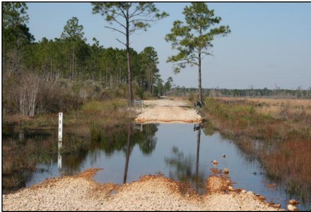
Figure 3. Low Water Crossing
