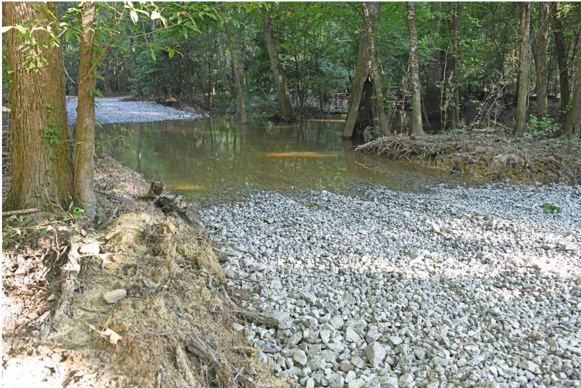
Post-construction (5/15/2019; Road Impediment to Natural Flows Removed)
