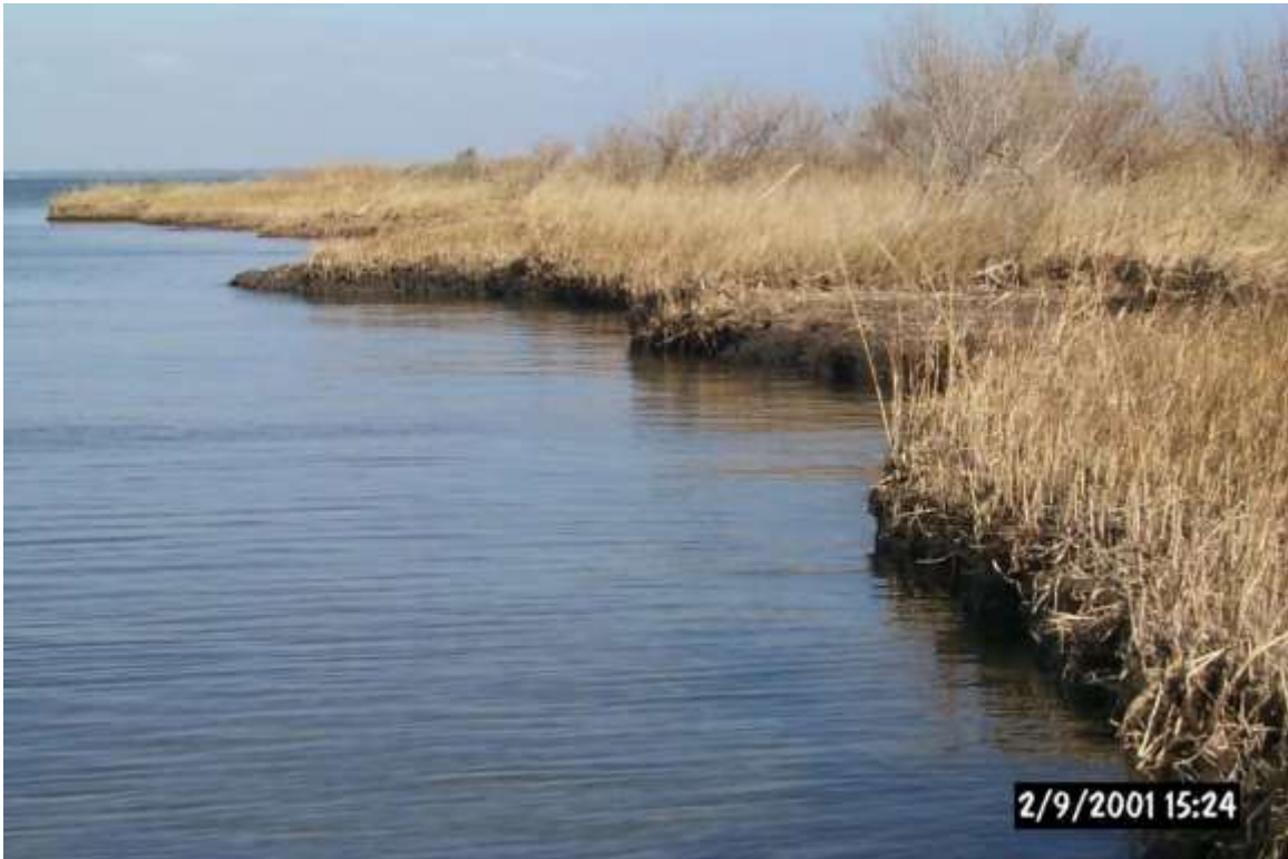
Figure 20. Live Oak Point, Undercutting of Salt Marsh (2/9/2001)
