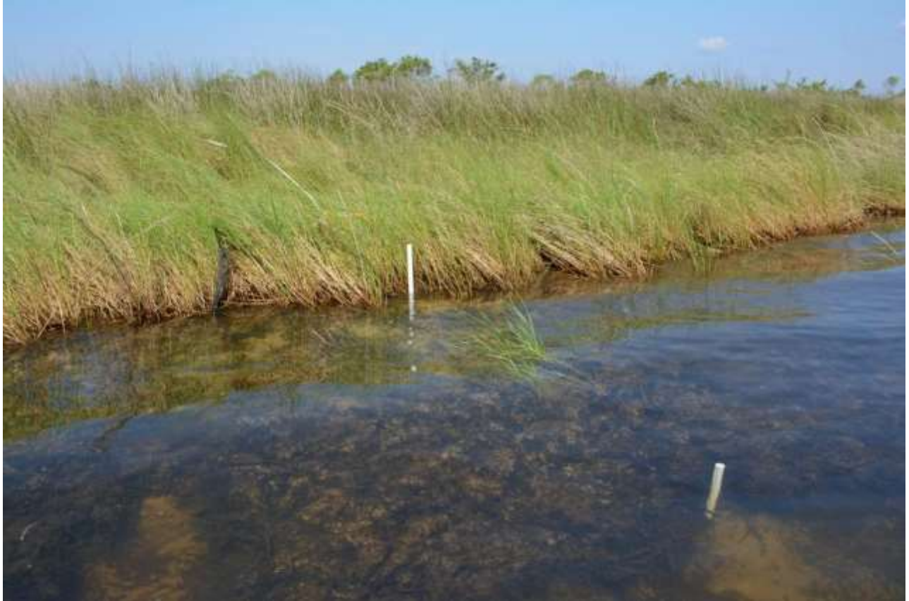
Figure 18. Undercutting of Salt Marsh (6/12/2019)
