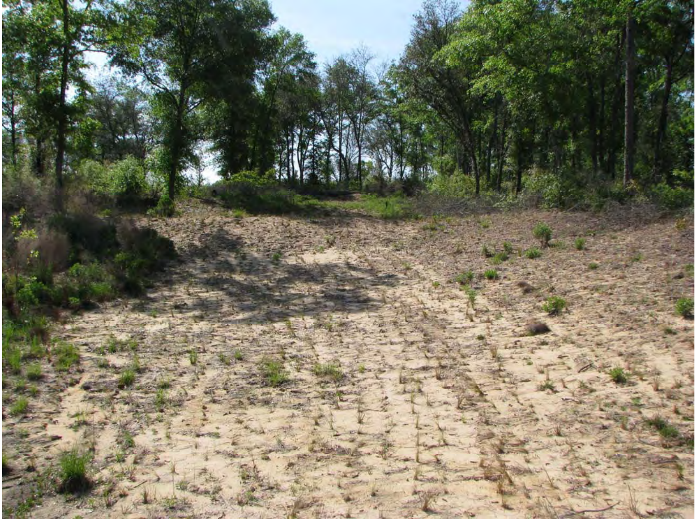
Re-planted Erosion Areas Showing Good Wire Grass Survival (040308)
