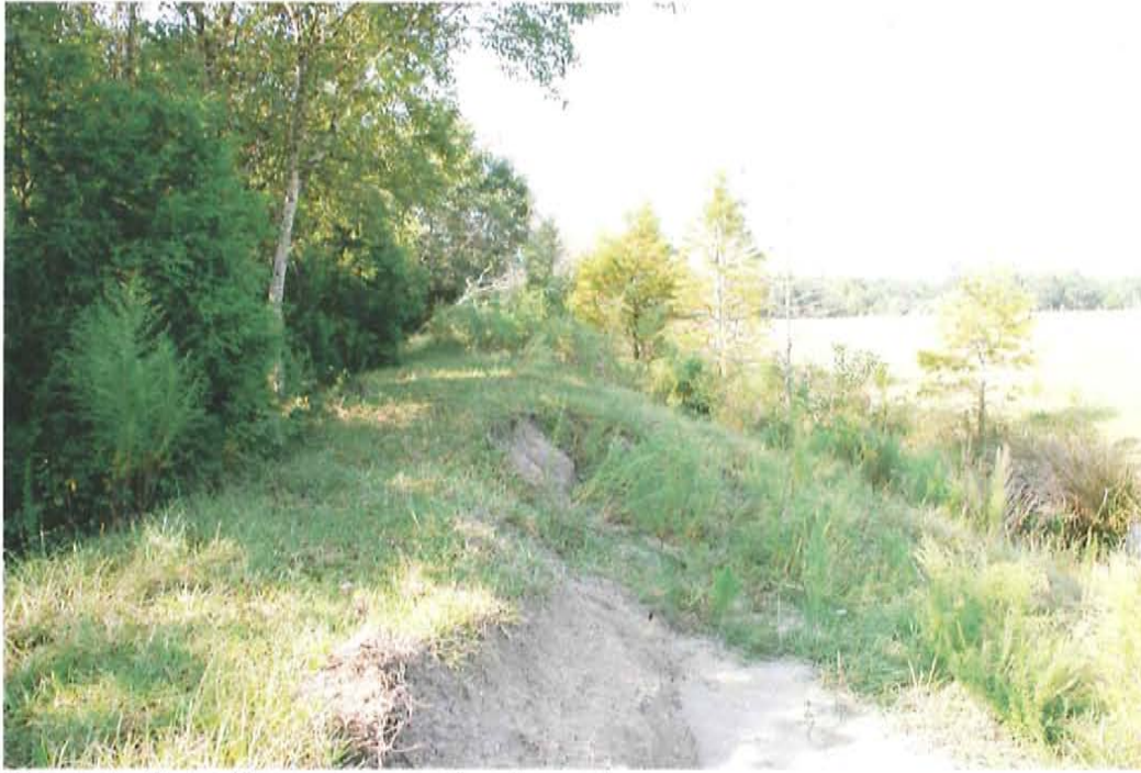
Figure 5. Top of berm surrounding the pasture
