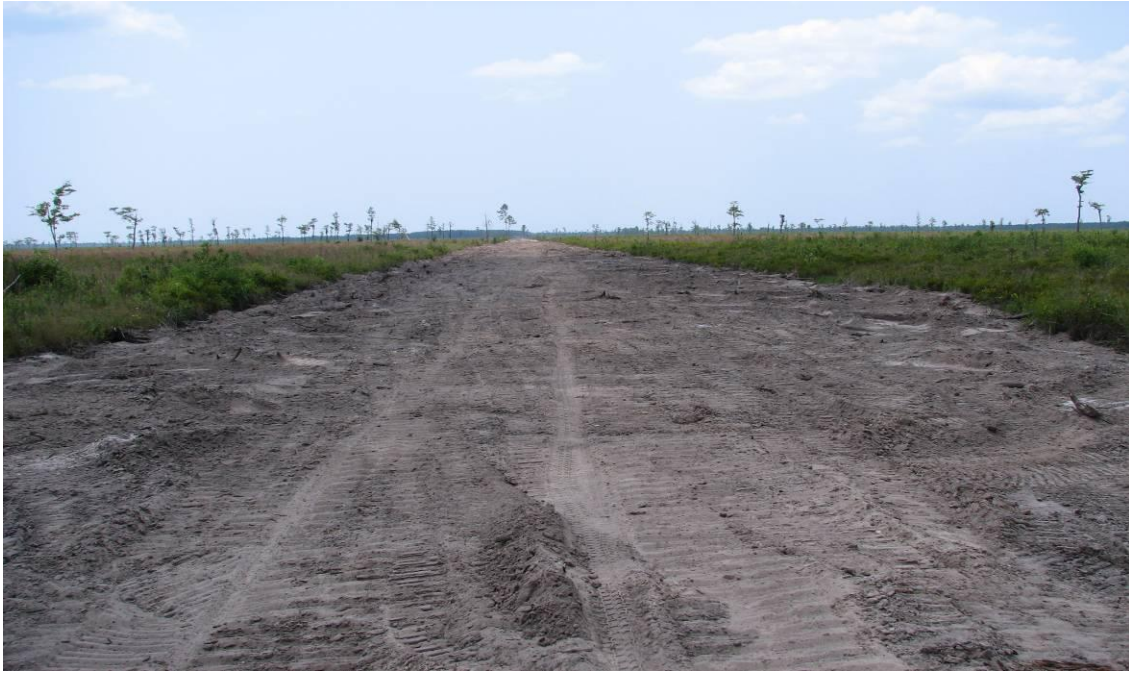
Figure 3. Road removal site #1 (westernmost road) after roadbed material was pushed into adjacent ditches and contoured to existing adjacent natural grade.
