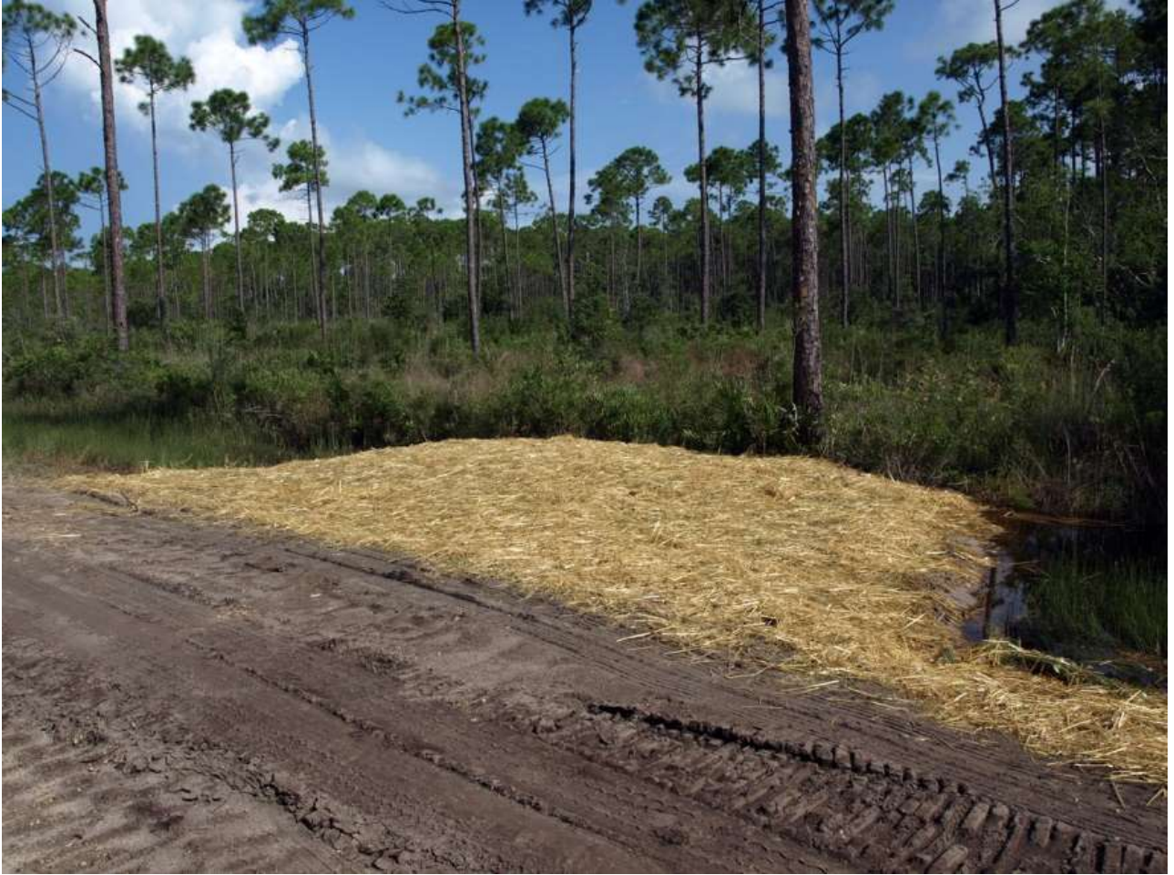
Typical Ditch Plug with Adjacent Hydric Pine Flatwoods in Background (9/3/2013)
