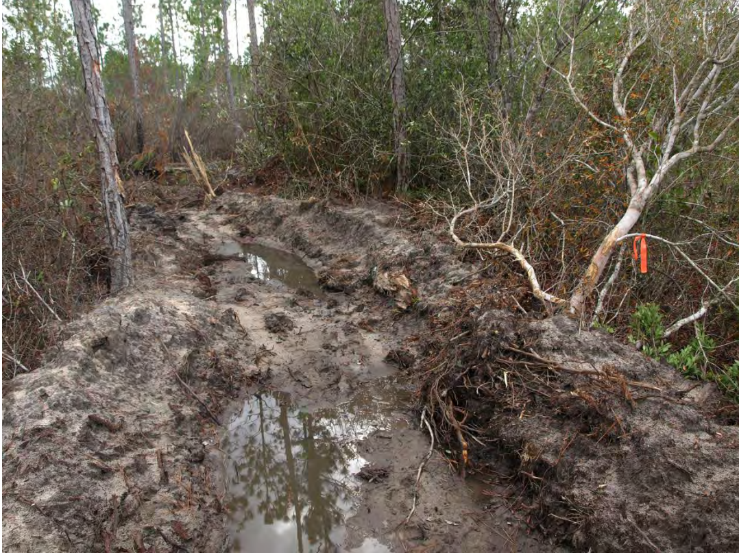
Photo 11. Plowed fire break. Photo point 12, facing north. 1/20/2012.
