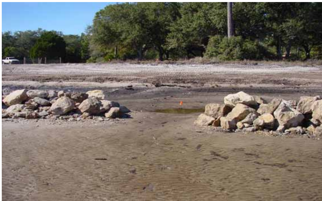
Figure 9. Close-up view of gap in breakwater (shown in center) to allow movement of water and organisms. Contoured shoreline with rubble removed seen in background.
