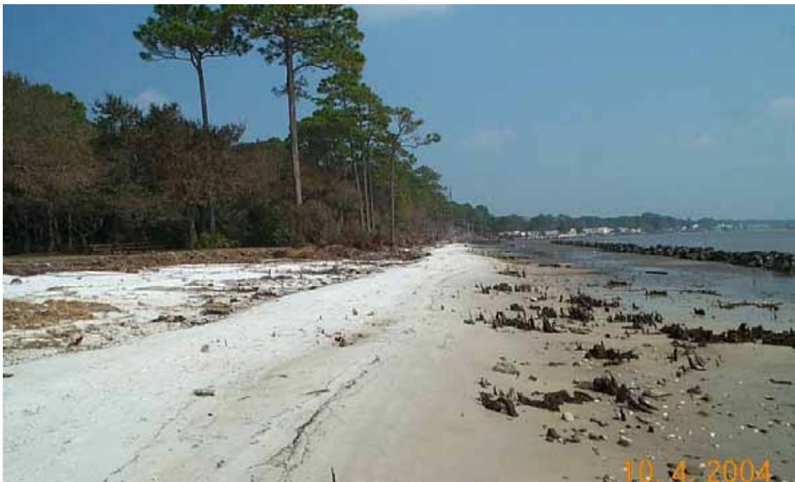
Figure 13. View of breakwater and adjacent eroded shoreline after Hurricane Ivan. Beach erosion was significant, extending at least 50 feet landward of previous beach/upland demarcation line.
