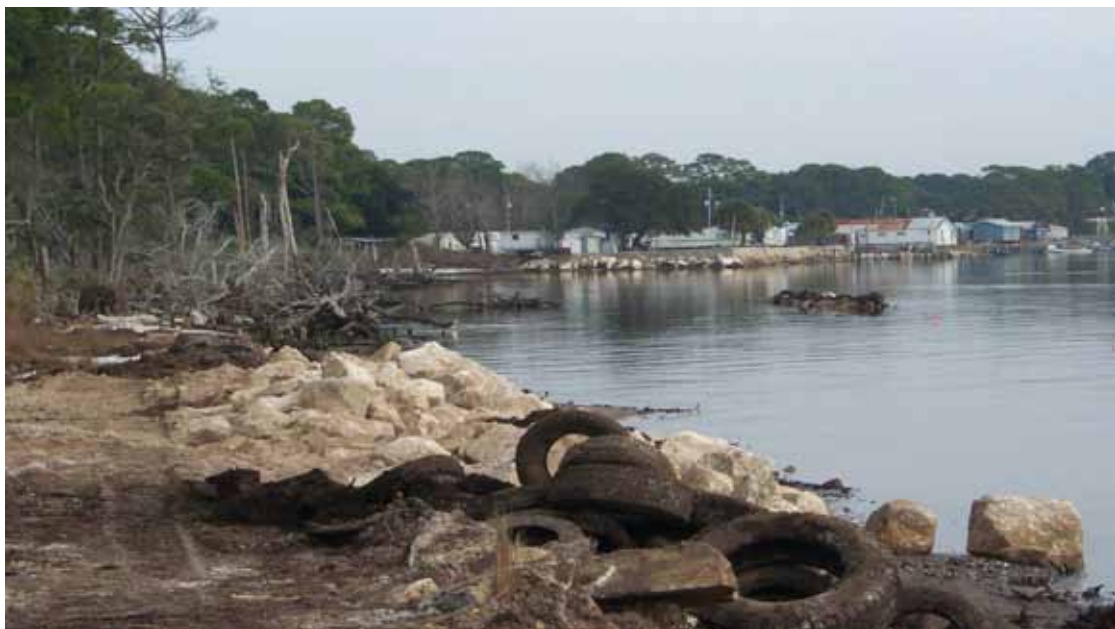
Figure 7. Cleanup of debris underway with old tires piled in foreground (later removed) and stone for breakwater just behind. The first section of breakwater is shown under construction in center right.
