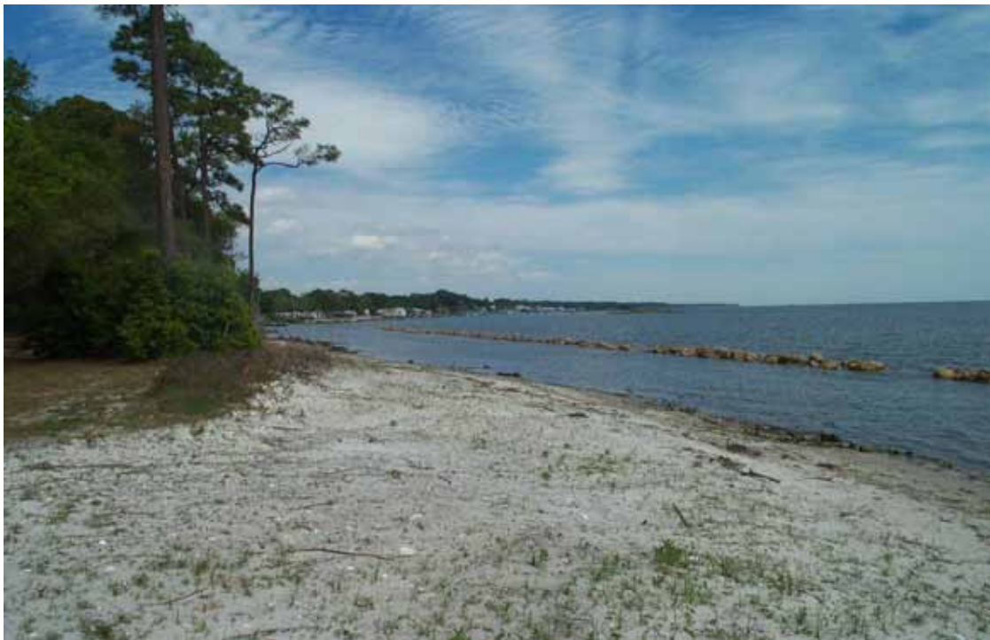
Figure 11. Post-construction view of breakwater showing rubble removed, shoreline contoured and initial recovery of beach vegetation.
