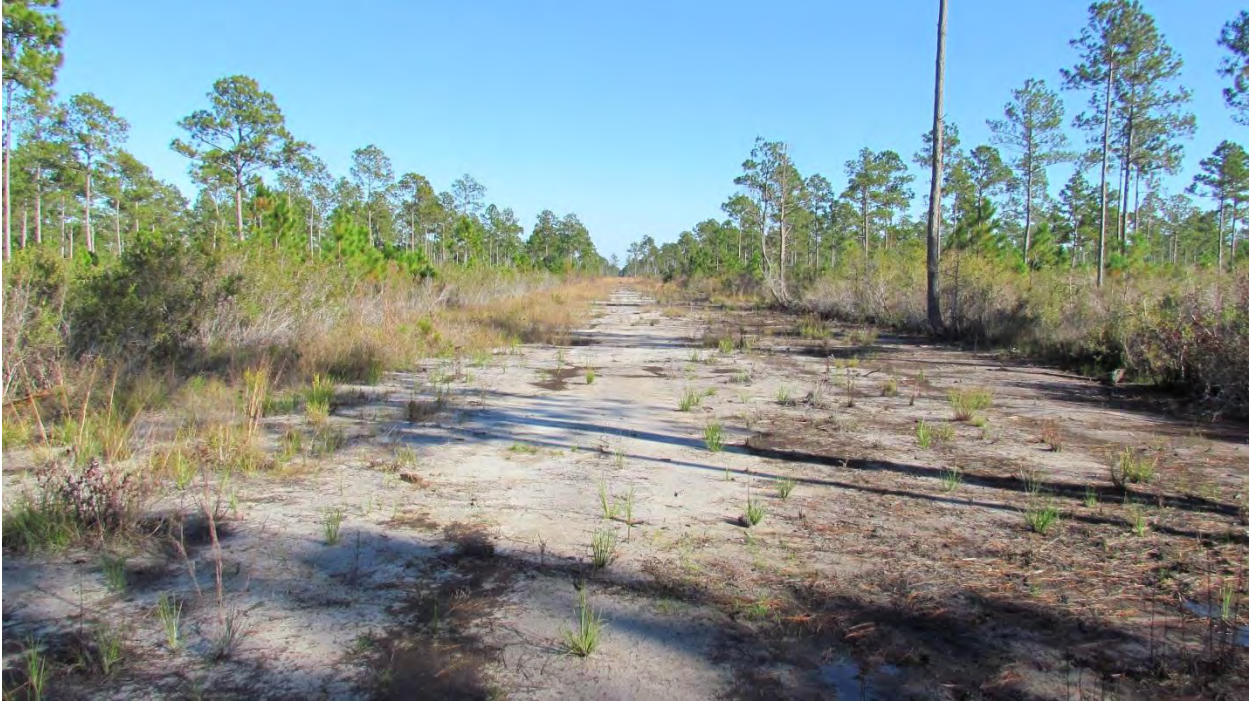
Photo 3. Whiskey George road removal with extensive patch of bare ground. Photo Point 4, looking east. 11/17/2011. RTN
