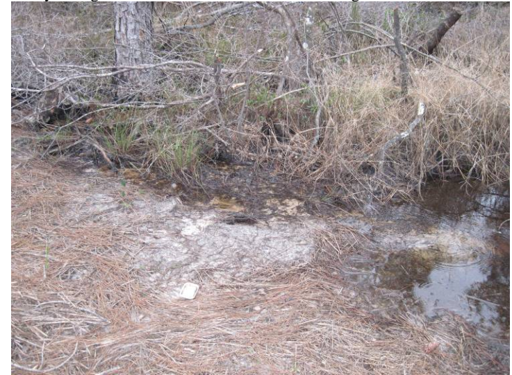
32. Whiskey George Tract. DB1. Water bypassing ditch plug
