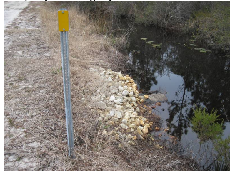
28. Whiskey George Tract. C2. North-facing culvert
