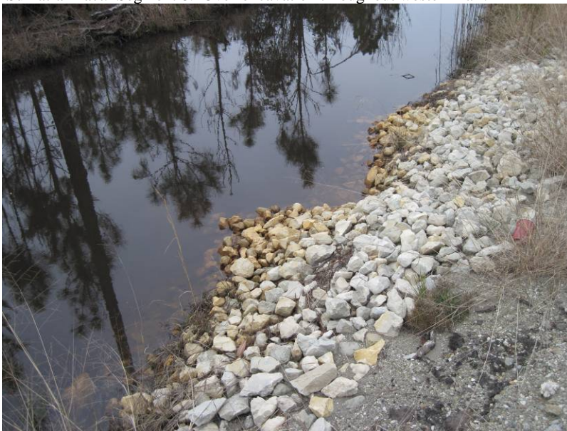
11. Sumatra Tract. Culvert Improvement – C4
