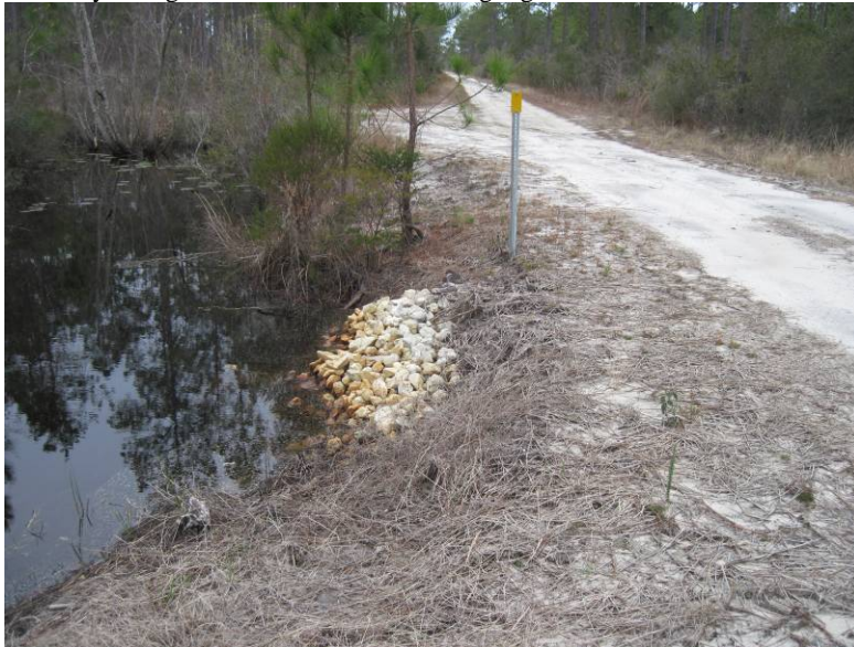
27. Whiskey George Tract. C2. South-facing culvert
