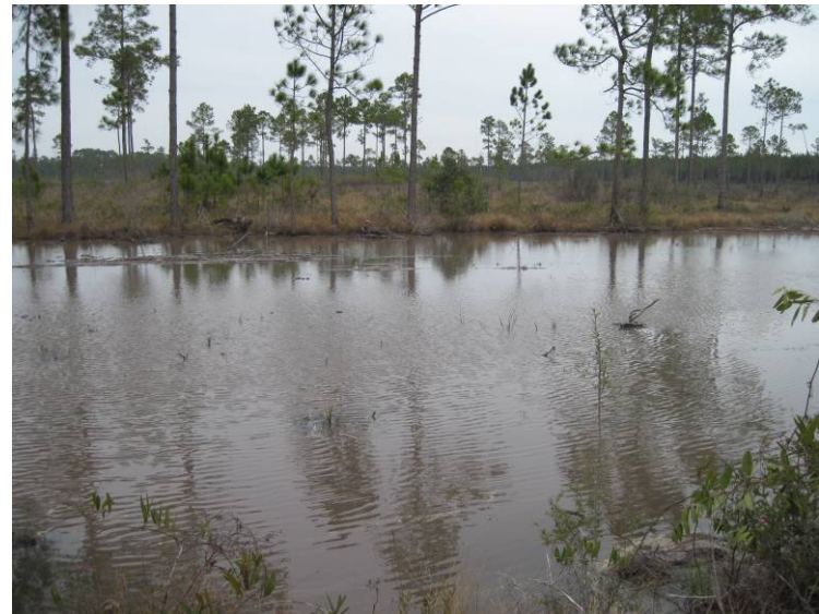
4. Sumatra Tract. Road Removal 16-3. Over-excavation
