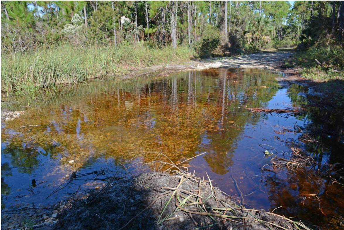
Post-construction (11/12/2015; Looking NNW)
