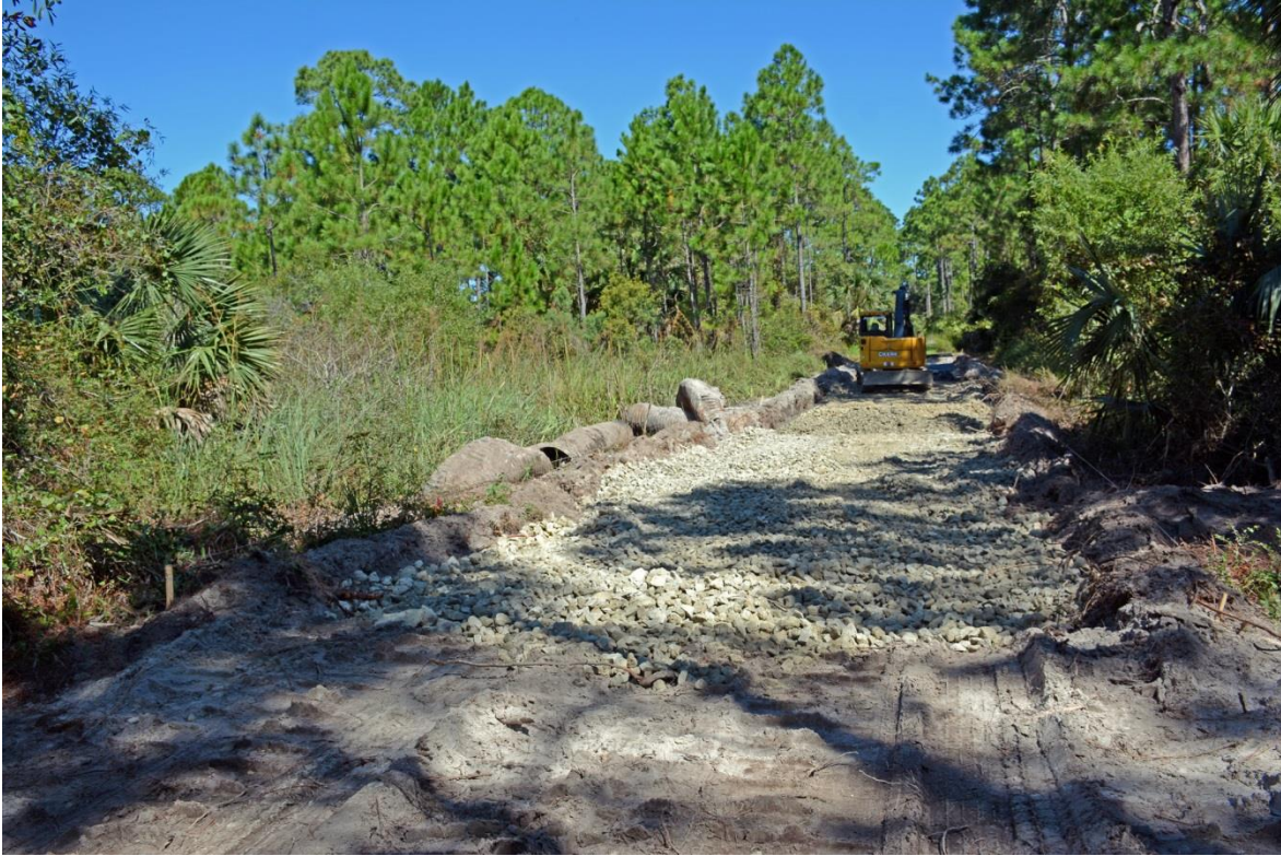
Construction (9/18/2015; Looking NNW)
