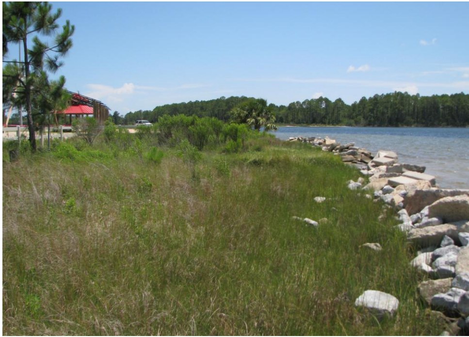
Southern restoration looking north (September, 2008)
