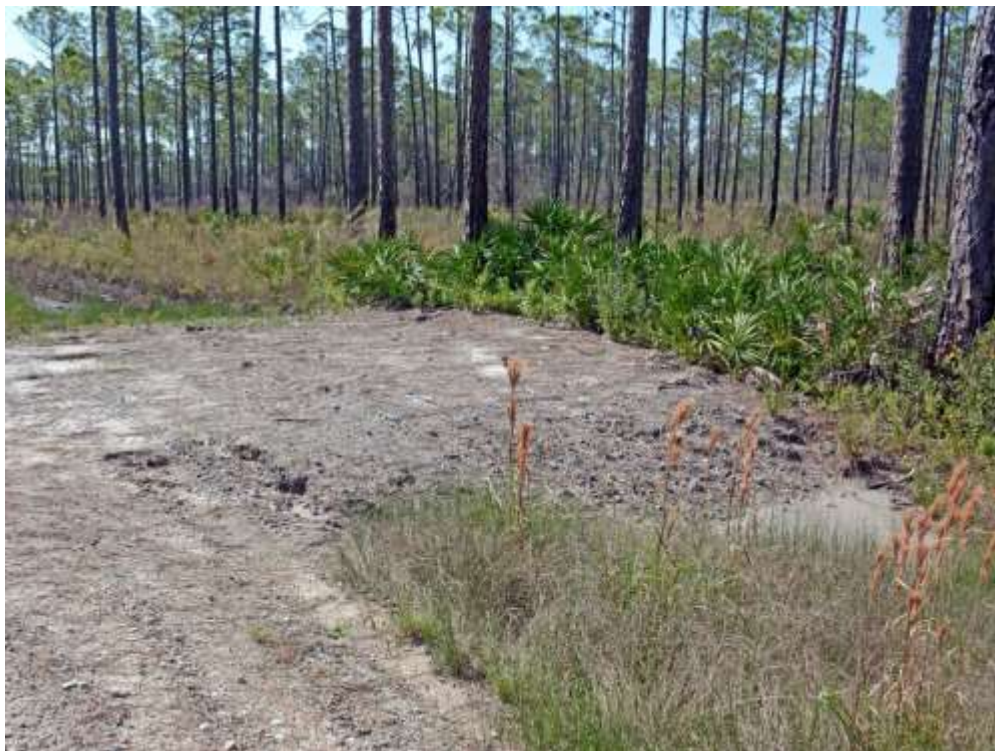
Typical Ditch Plug with Adjacent Hydric Pine Flatwoods in Background (4/8/2015)
