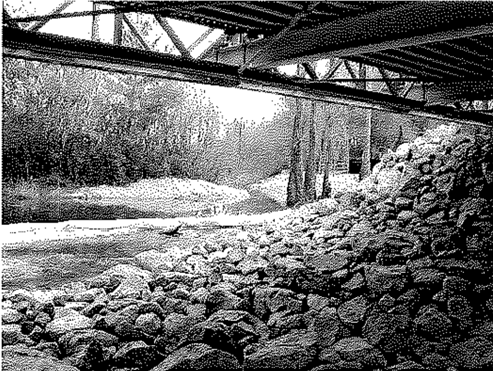
Bridge Construction at Greenhead Branch (February 2007)
