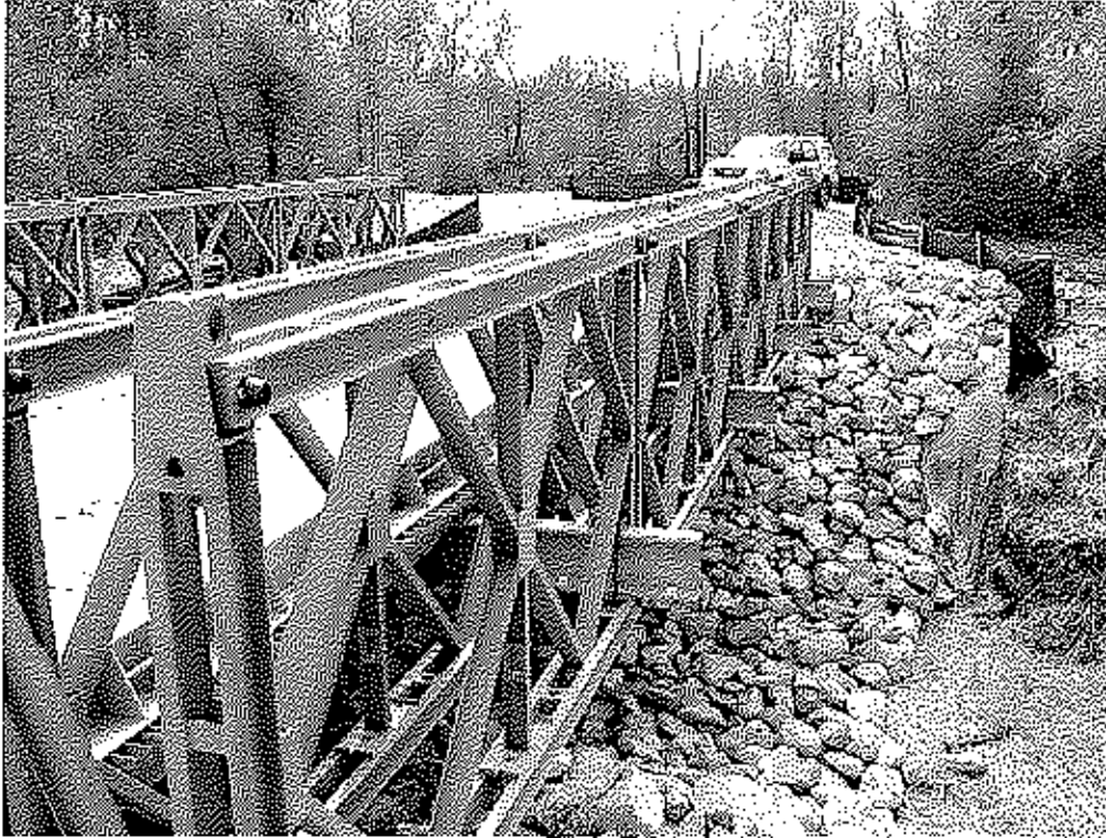
Bridge Construction at Greenhead Branch (February 2007)
