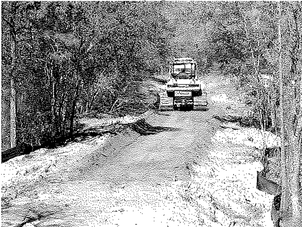
Roadfill Removal Between Little Deep Edge and Greenhead Branch (March 2007)
