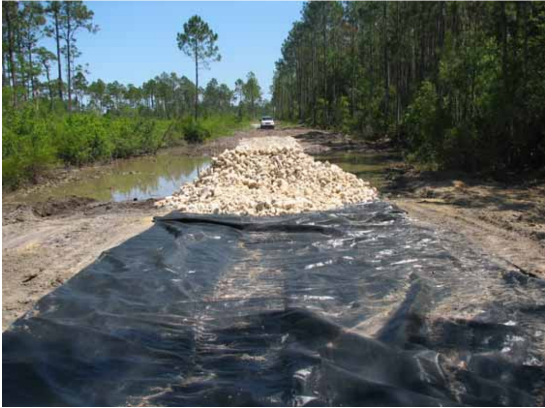
Low-Water-Crossing Construction
