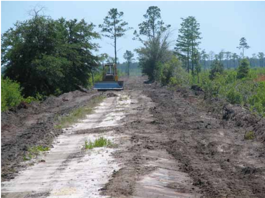
Removal of Road and Ditch
