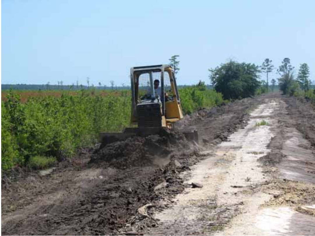
Removal of Road and Ditch
