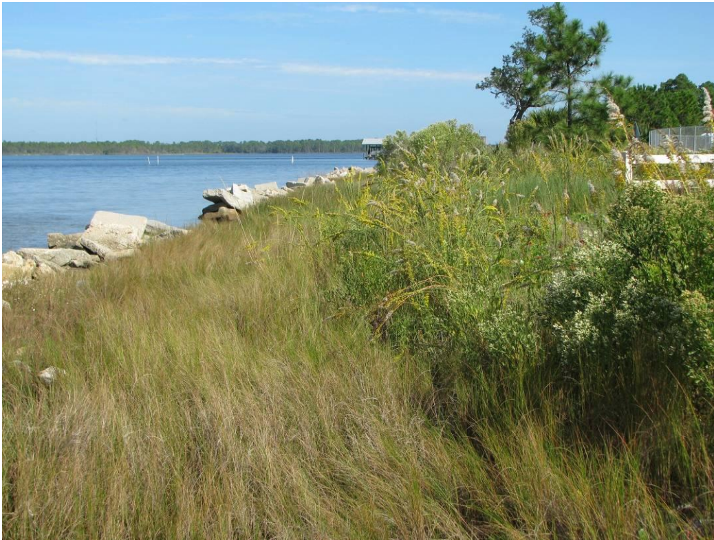
Southern restoration looking south (October 30, 2009)
