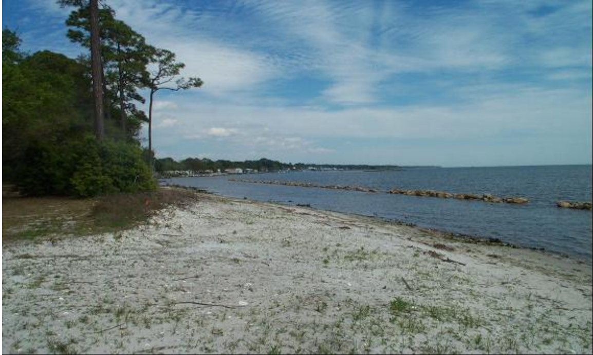
Figure 4. Post-construction view of breakwater showing rubble removed, shoreline contoured, and initial recovery of beach vegetation (June 2004).
