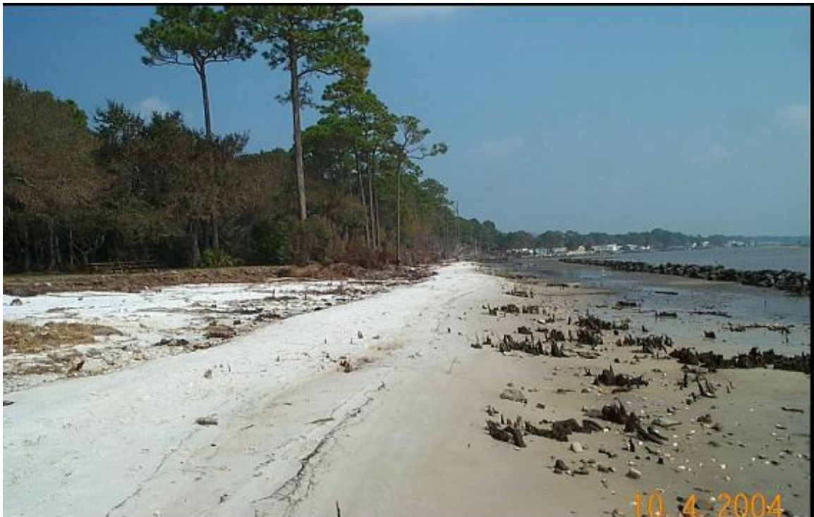
Figure 5. View of breakwater and adjacent eroded shoreline after Hurricane Ivan (September 2004). Beach erosion was significant, extending at least 50 feet landward of previous beach/upland demarcation line.
