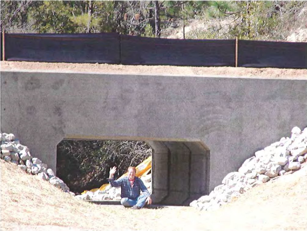
Culvert Construction at Powerline Pond (March 2007)
