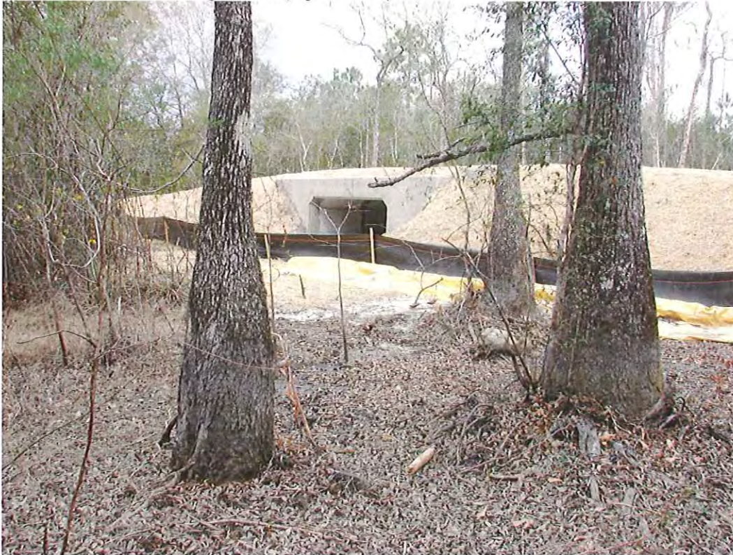
Culvert at Old Pine Log Creek (April 2007)
