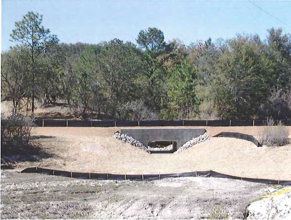
Culvert Construction at Powerline Pond (Pond Near Dry) March 2007
