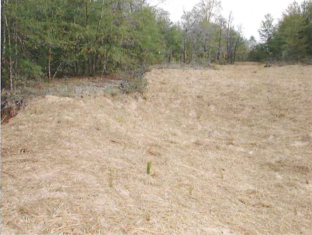
Erosion Control Site #7 at Greenhead Branch March 2007
