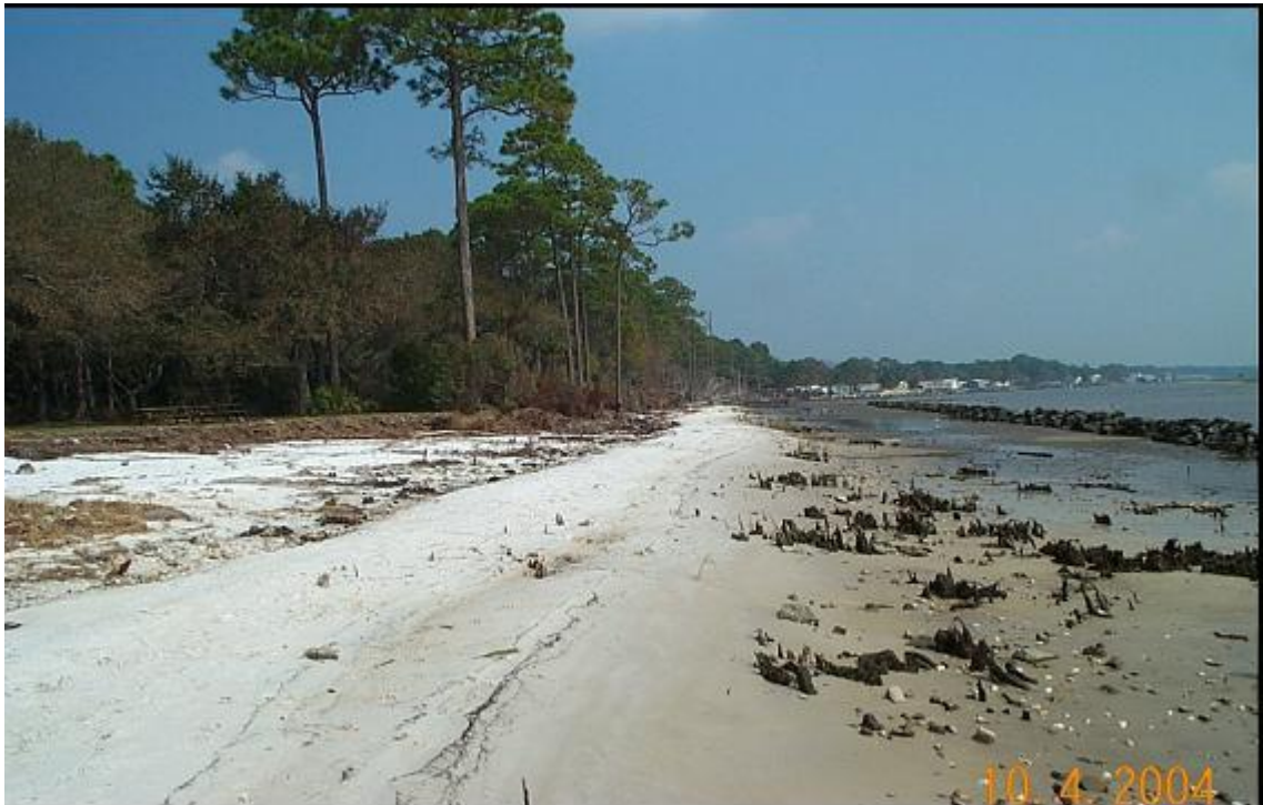
Figure 5. View of breakwater and adjacent eroded shoreline after Hurricane Ivan (September 2004). Beach erosion was significant, extending at least 50 feet landward of previous beach/upland demarcation line.
