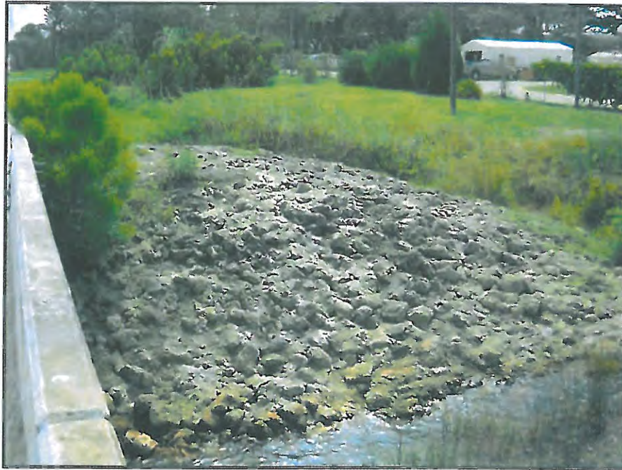
Photograph 3 – South side of East approach (facing East)
