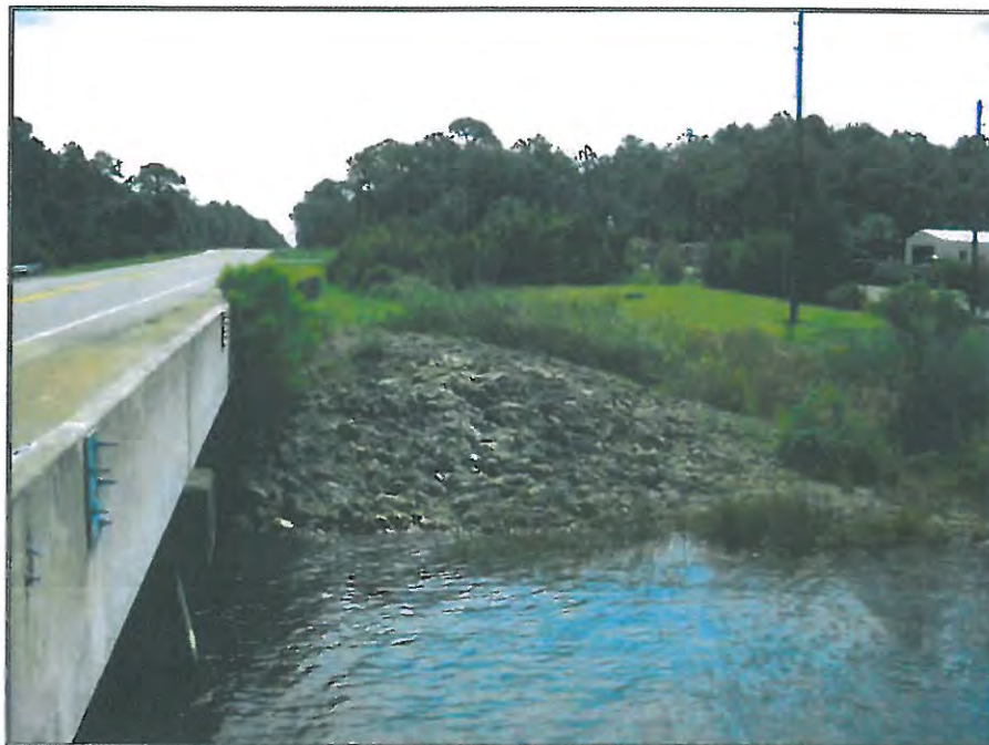
Photograph 4 – South side of East approach (facing East)
