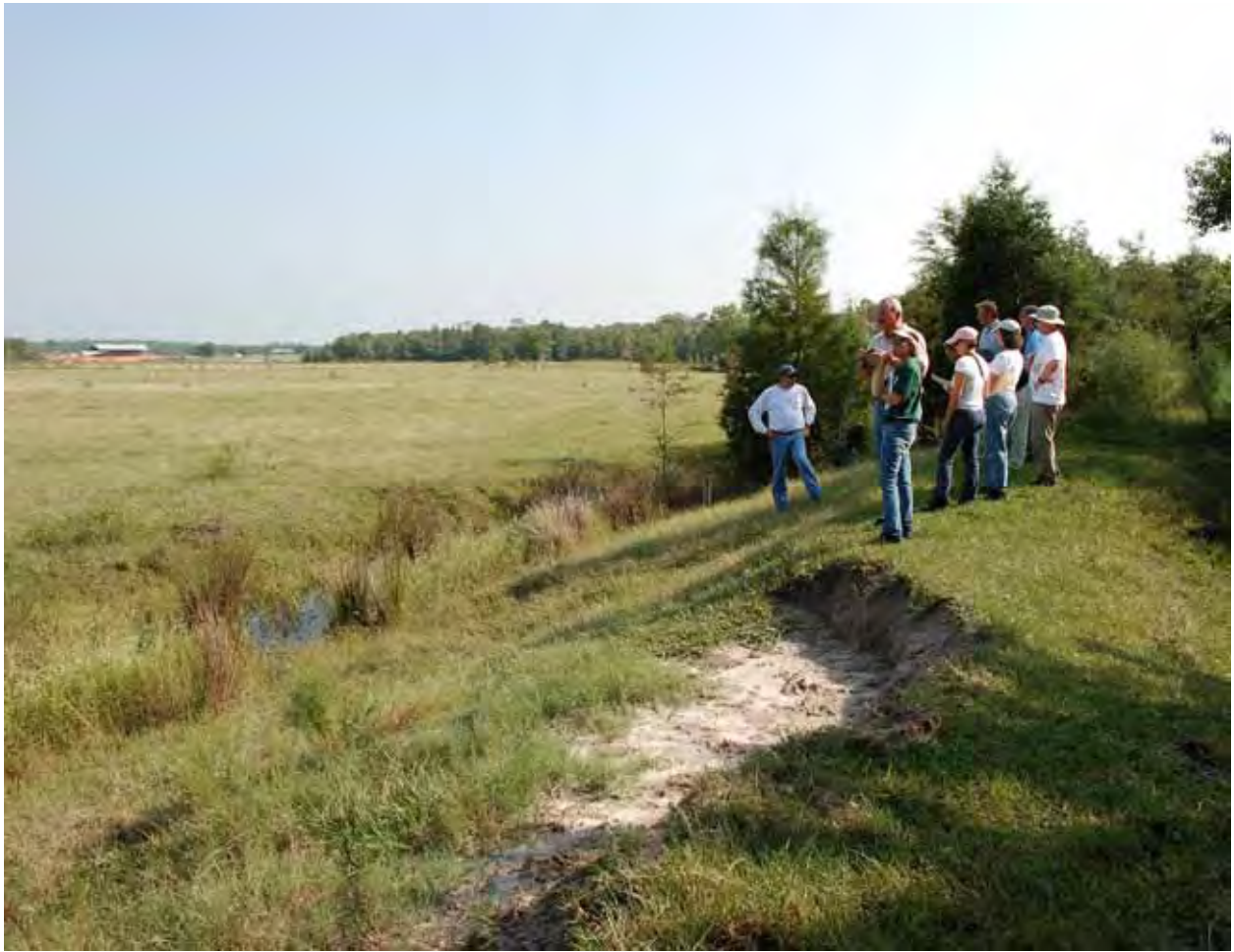
CORPS / MRT inspecting Yellow River Ranch pasture and dike (9/25/07)
