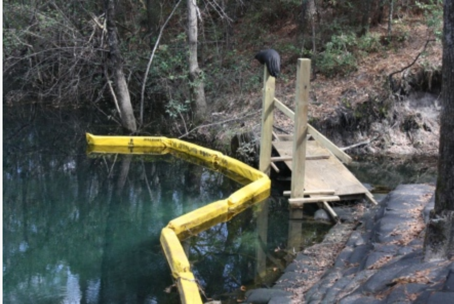
Devil's Hole spring is currently closed for the restoration project.
