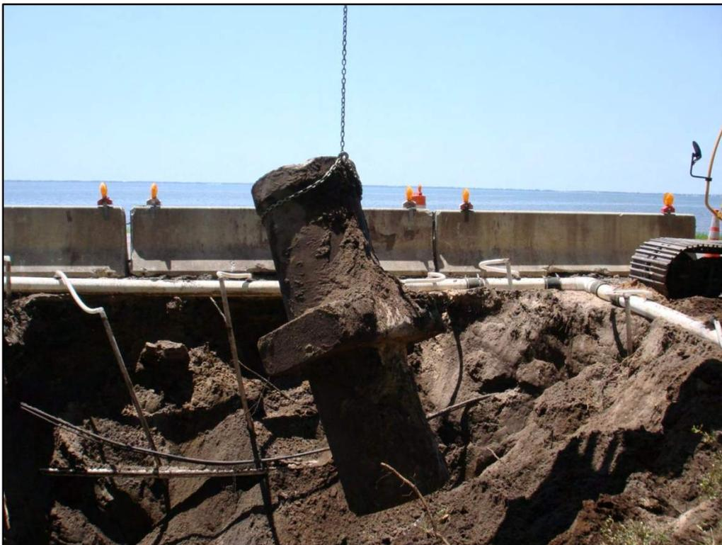
Figure 38: Site 6 - Concrete Collar Removal
