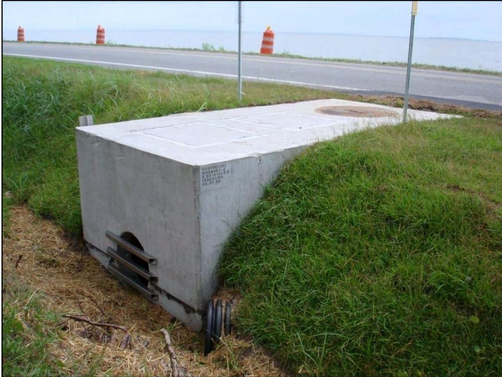
Figure 41: Site 6 – Completed Installation With Safety Bars
