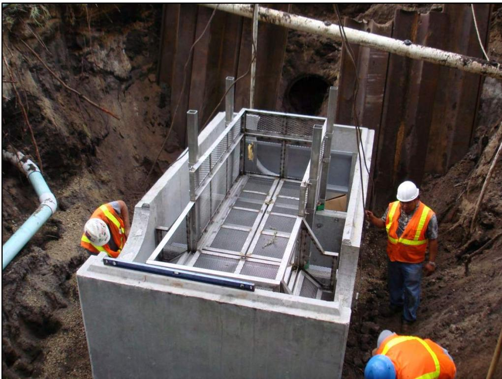
Figure 33: Lower Section Placement
