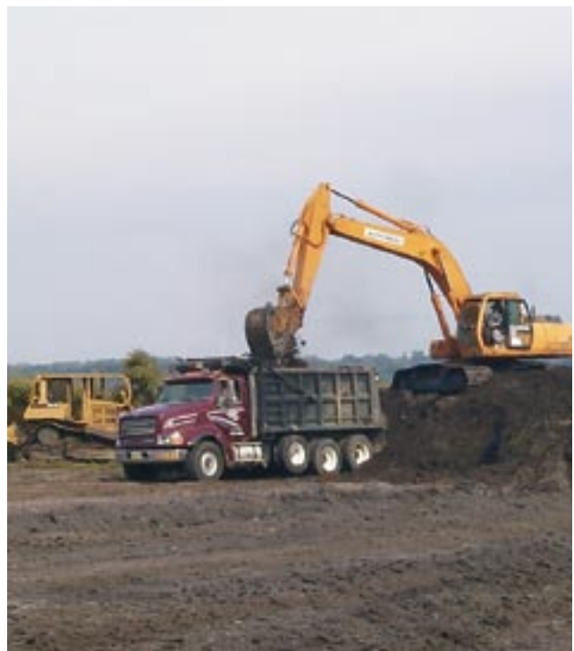
LAKE JACKSON RESTORATION
