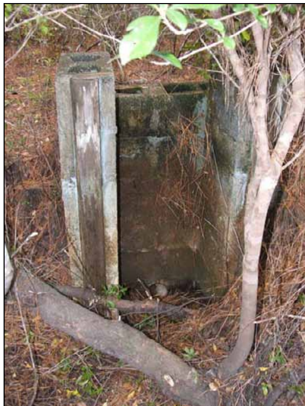
Figure 100. Example of water-control device remnants along Carter's canal along the west side of Dykes Mill Pond.
