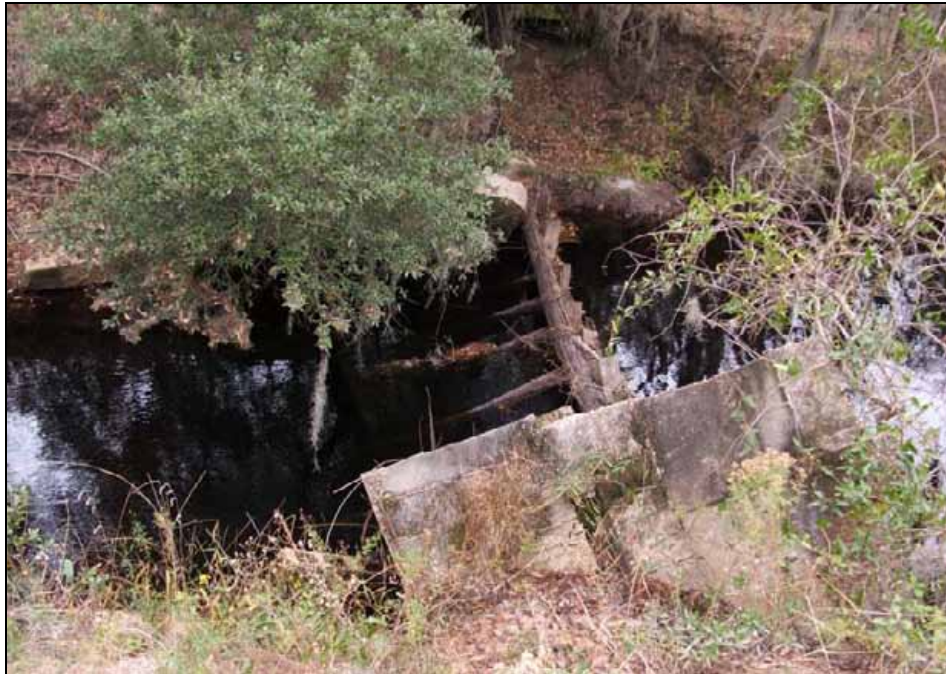
Figure 102. Photograph of the 8WS1031 water-control gate remnants at Black Pond.
