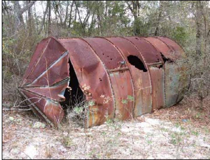
Figure 61. Photograph of the water tank located northwest of 8WS469, view to the northeast.
