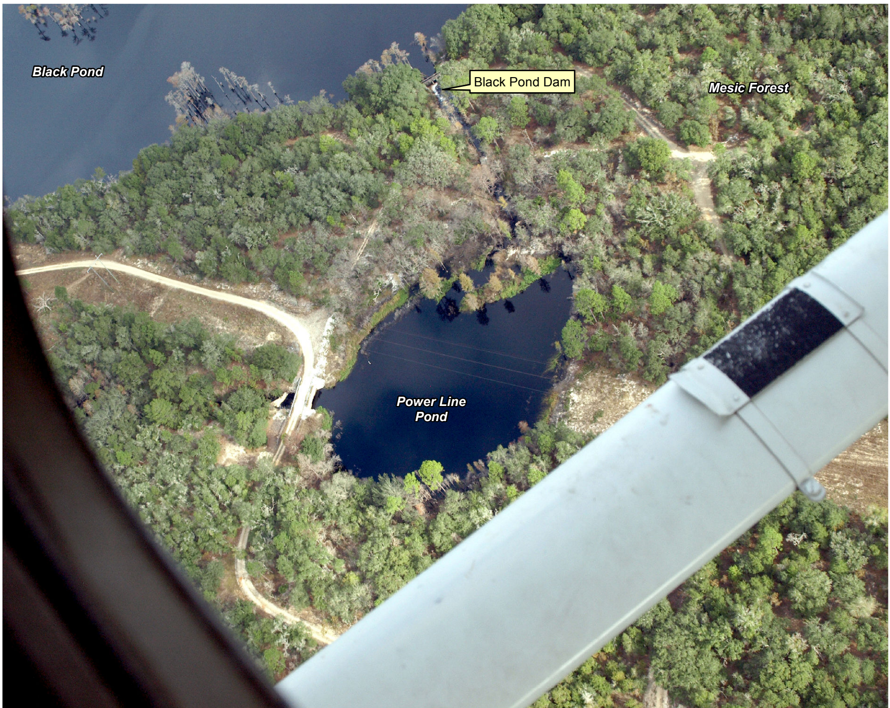
Sand Hill Lakes Mitigation Bank, Oblique Aerial, Looking Approximately North, 11/20/2013 (Photo #88)
