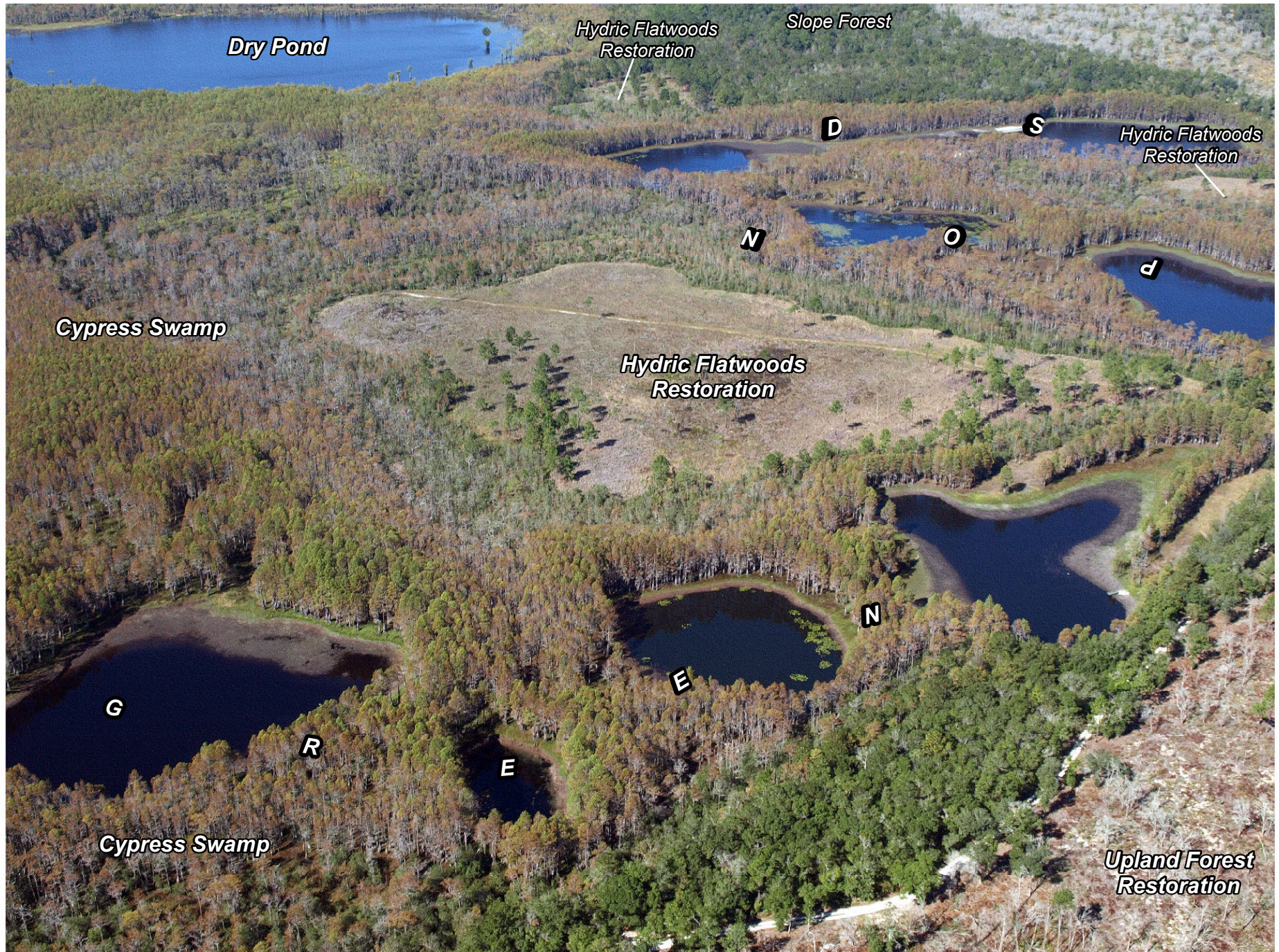
Sand Hill Lakes Mitigation Bank, Oblique Aerial, Looking Approximately West, 10/14/2011
