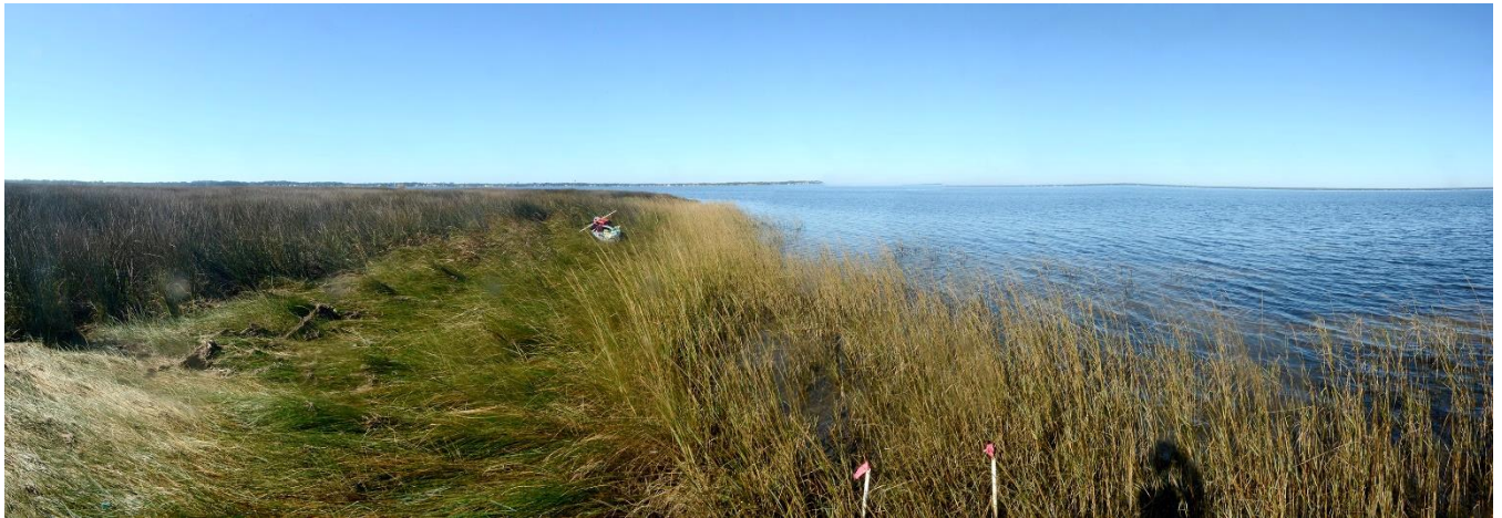
Figure 22. Photo Point T9 Looking West – 11/8/2021
