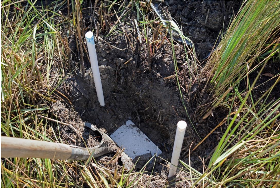
Figure 29. Installation of Sediment Accretion Monitoring Point
