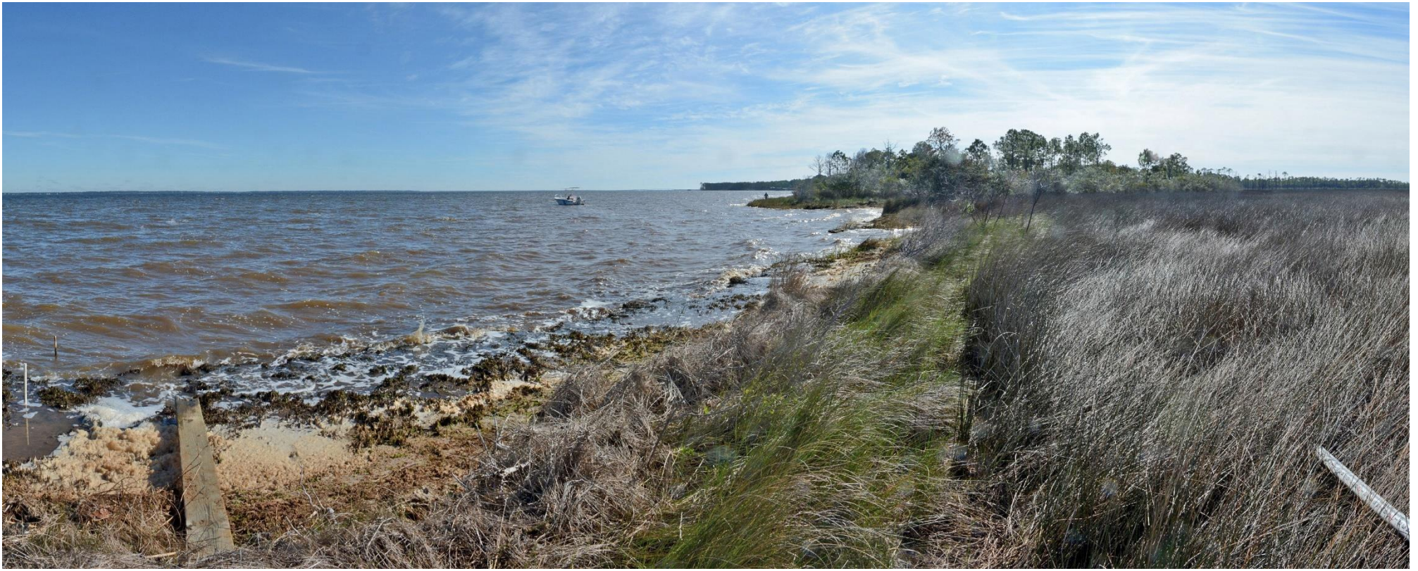
Photo Point A3 – 1/30/2020 (Looking Approximately Southeast)
