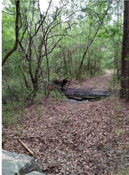
Low-Water Crossing on Middle Road
