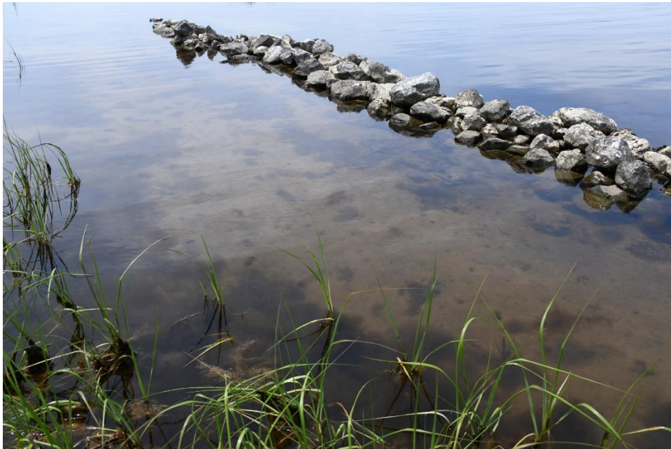
Figure 32. Sediment Accumulation Behind Constructed Breakwaters (5/3/2024)
