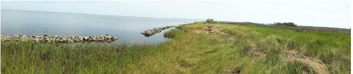
Figure 21. Project Site Photo Point T6 Looking East – 5/3/2024
