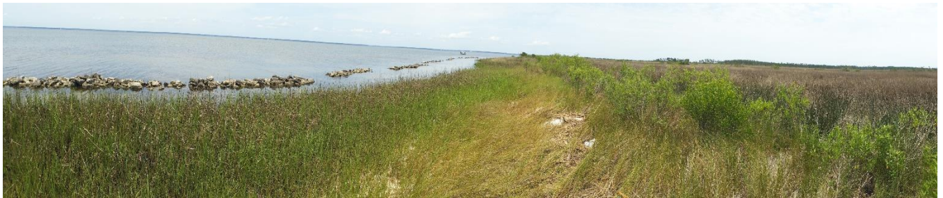
Figure 17. Project Site Photo Point T4 Looking East – 5/3/2024
