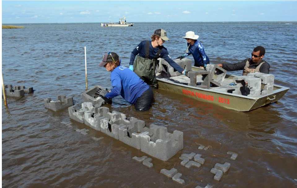
Figure 23. Breakwater Construction Using "Oyster Castles" (11/13/2024)
