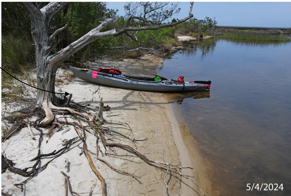
Figure 29. Washout of Planted Vegetation Not Protected by Breakwaters
