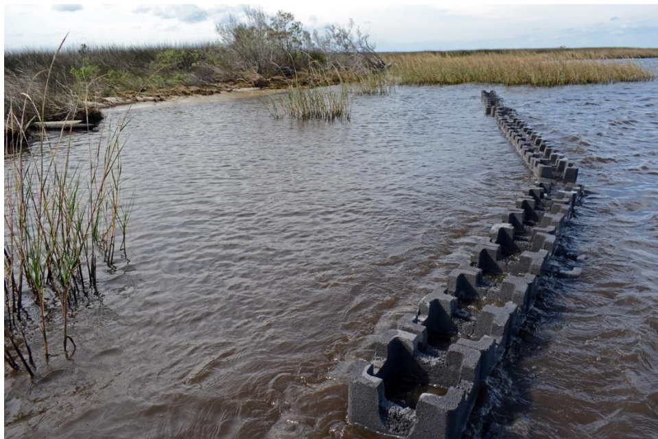
Figure 24. Newly Constructed Breakwater Segment Using "Oyster Castles" (11/13/2024)
