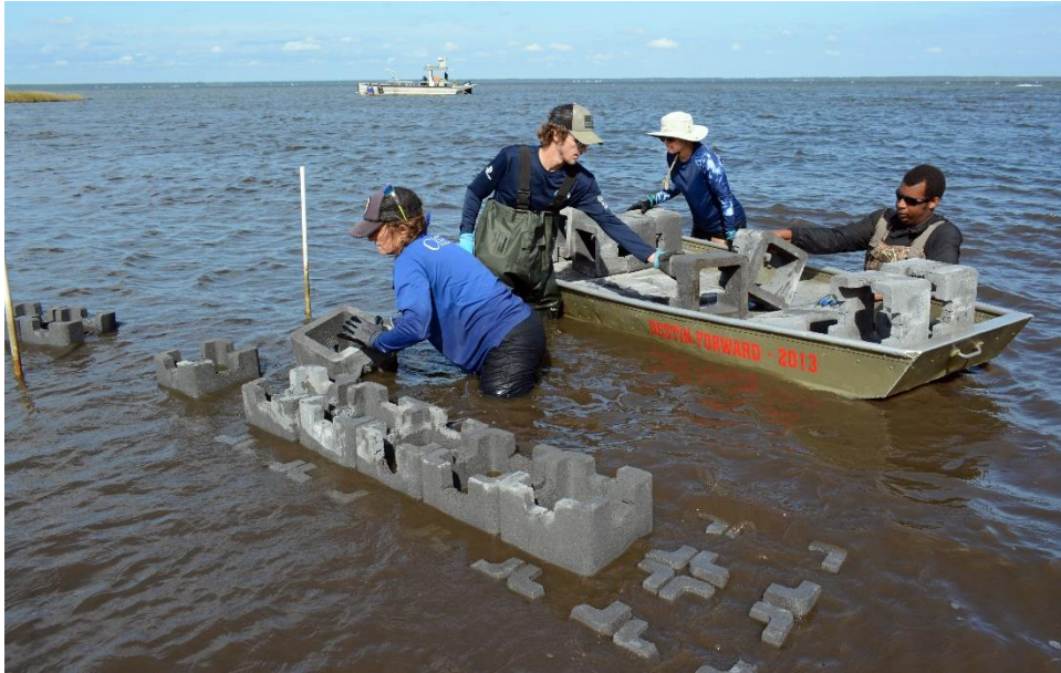
Figure 23. Breakwater Construction Using "Oyster Castles" (11/13/2024)
