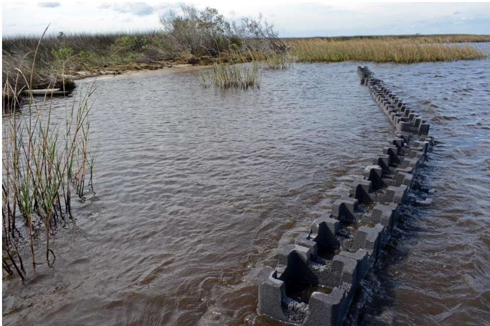
Figure 24. Newly Constructed Breakwater Segment Using "Oyster Castles" (11/13/2024)
