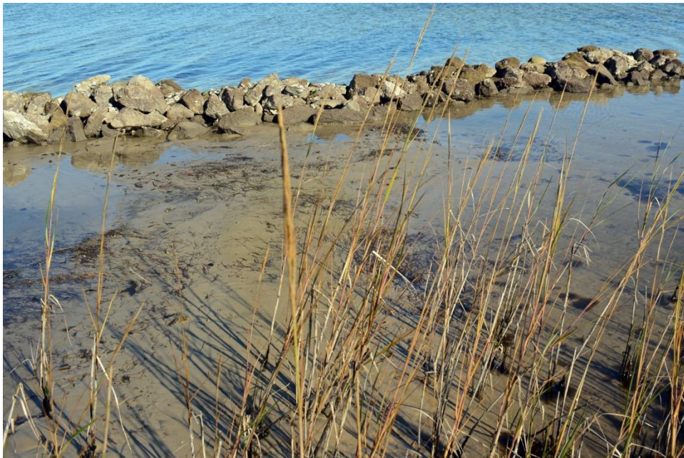
Figure 28. Sediment Accretion Behind Limerock Breakwater (12/16/2024)
