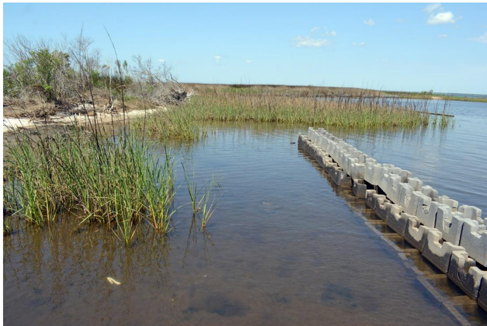
Figure 25. Recent Breakwater Construction Using "Oyster Castles" (4/11/2025)
