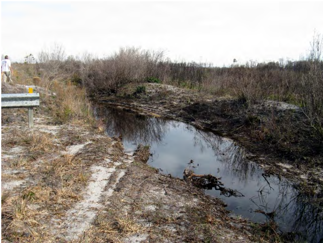
Photo 4. Western end of road removal Segment 1 indicating loss of ditch plug and possible vehicle tracks bypassing the guard rail and entering the site; taken at photo point 2 looking SE, 1/18/12. RTN
