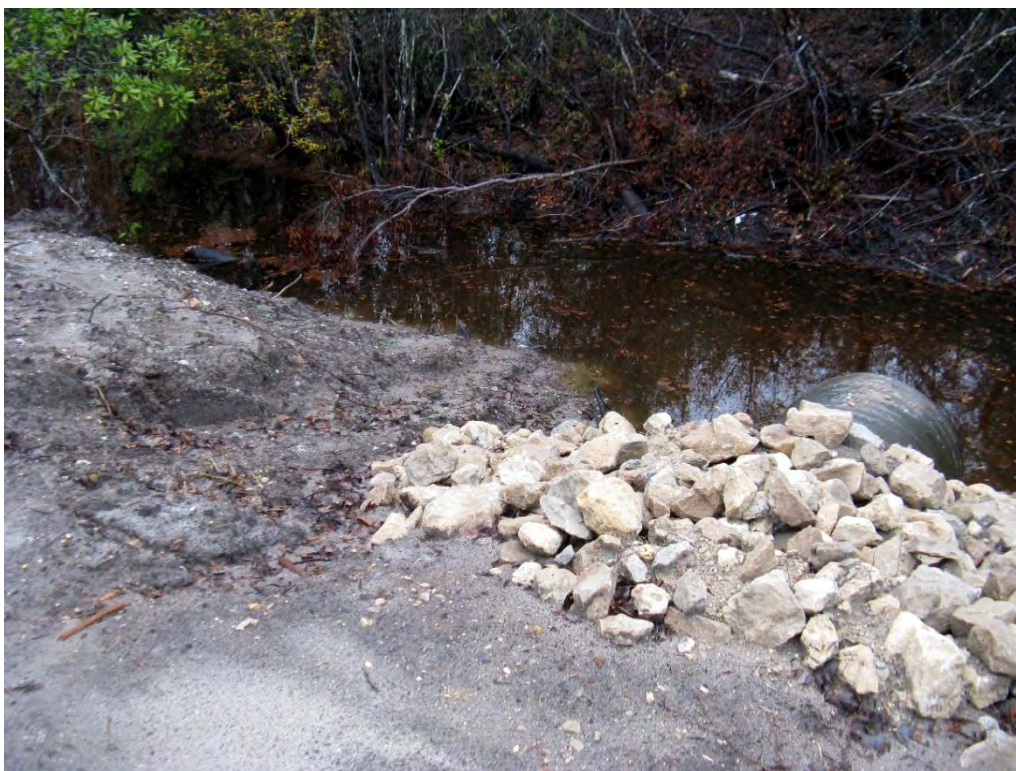
Photo 10. Minor erosion around side of newly installed culvert (e.g., C10); taken at photo point 9, 1/18/12.
