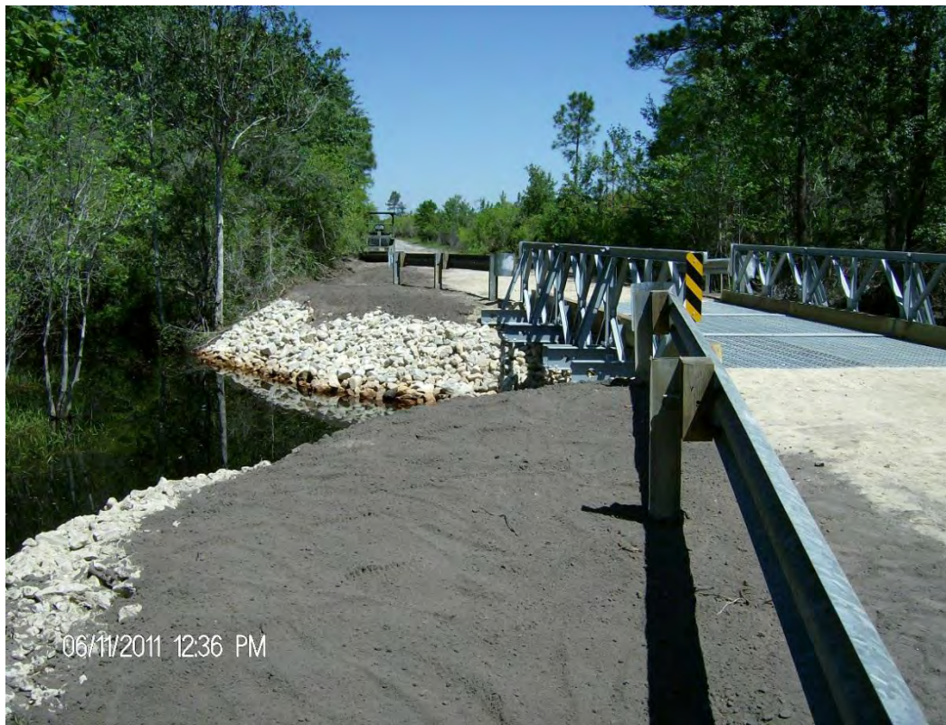
Photo 12. Three-span Bailey bridge over a tributary of Pine Log Creek; taken at photo point 11, 6/11/11. RTN
