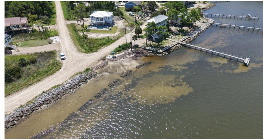
OysterCorps Shoreline Stabilization, St. George Island
