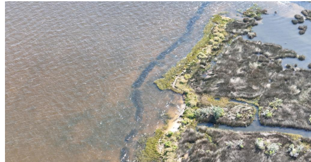
Live Oak Point Oyster Breakwater
