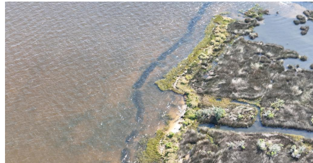
Live Oak Point Oyster Breakwater
