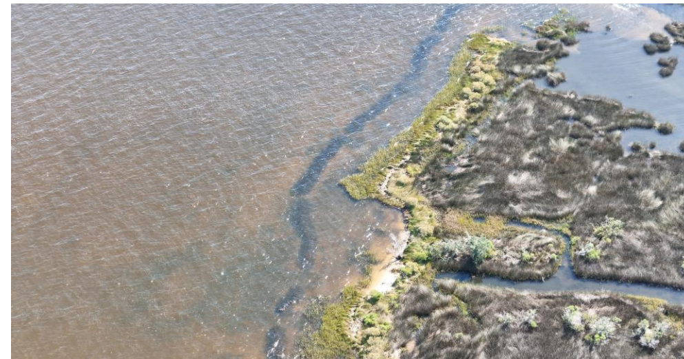
Live Oak Point Oyster Breakwater
