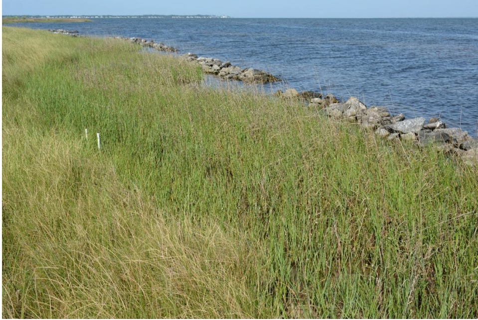
Figure 40. Marsh Expansion Behind Breakwaters
